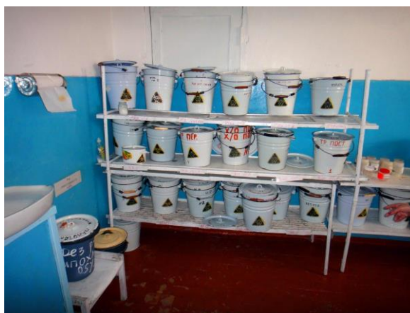
Photo 2: On a daily basis the infectious waste is removed from the wards and taken to a central storage close to the treatment area. Enamel containers are used to hold the waste, as this is an inexpensive solution. Each hospital department have their own designated buckets.
