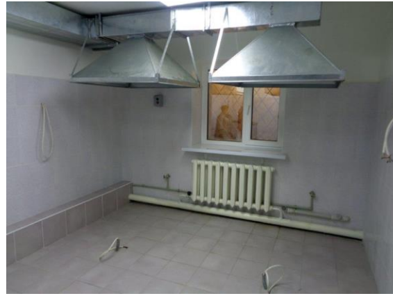
Photo 6: A future autoclaving room with the ventilation hoods in place.
